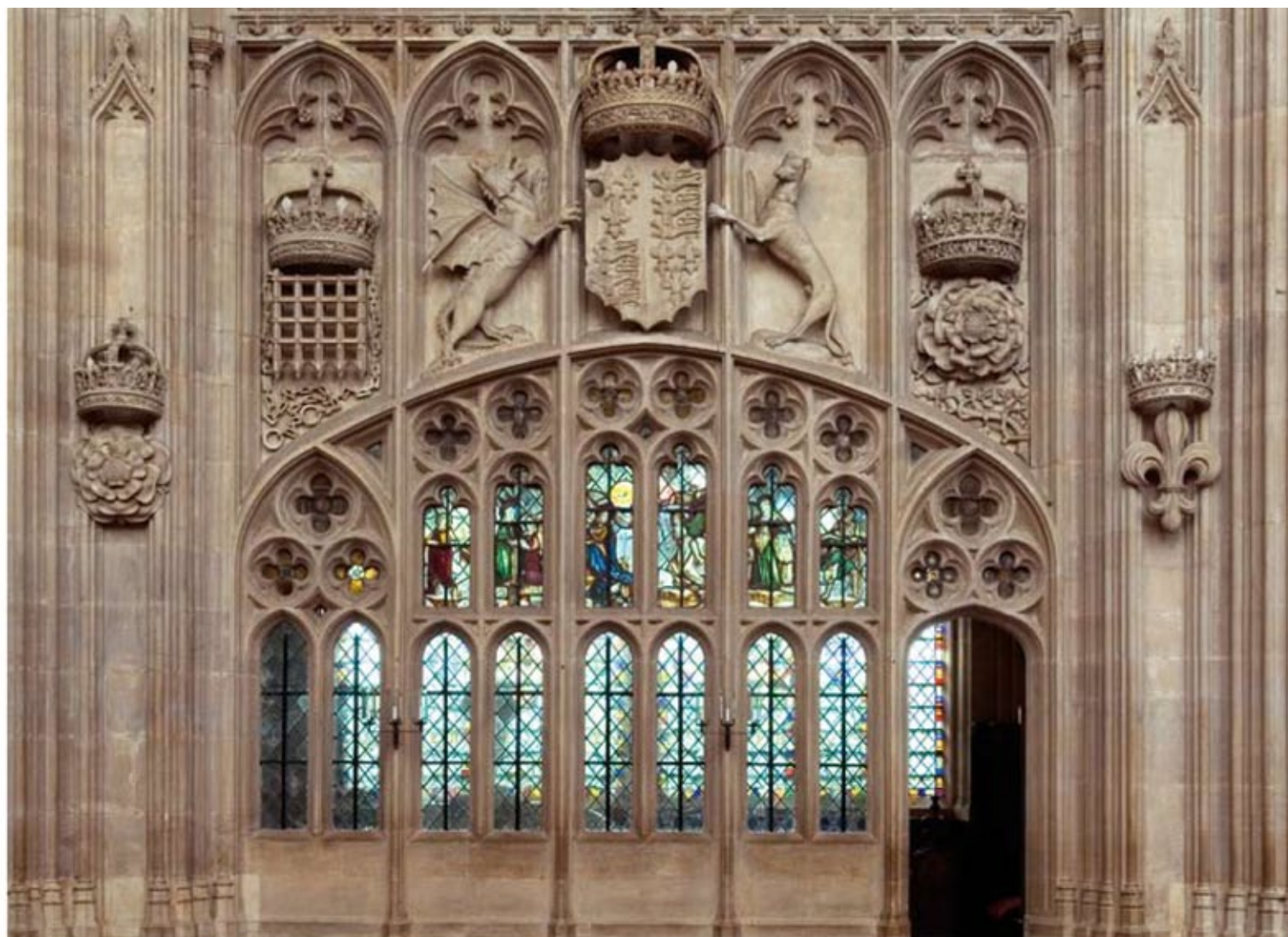
↑ Fig 6: The side chapels in the nave are separated from the main space by elaborate screens of tracery. Within the panelling are suspended massive heraldic sculptures, including the arms of England with supporters and the crowned emblems of the Tudor dynasty: roses, fleurs-de-lis and portcullises. Wastell's rich detailing is brilliantly integrated within the constraints imposed by the fabric he inherited
