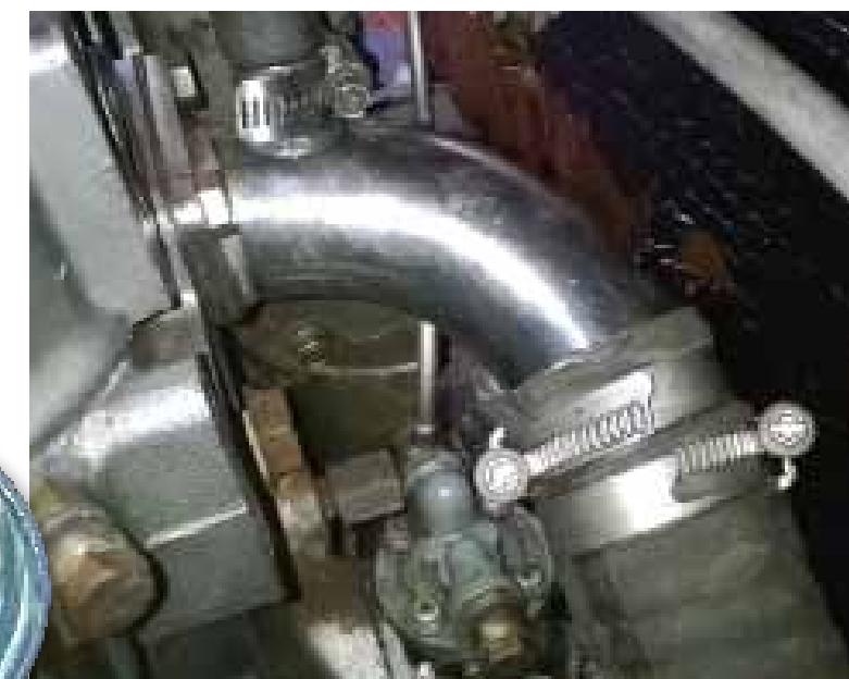
The new elbow should be fitted to the engine with a new gasket, all hoses reattached and the hose clips done up. The engine should be run to check for water and exhaust leaks
