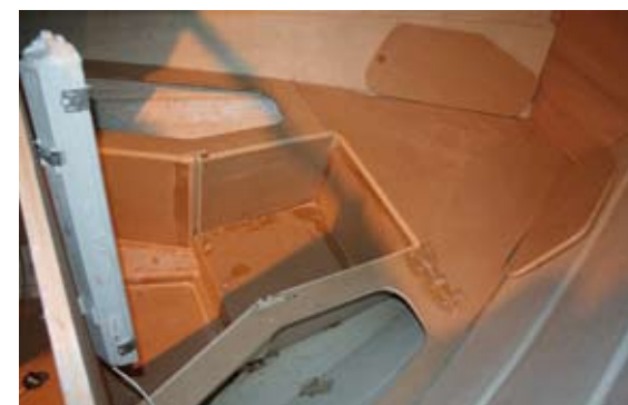
Life at the sharp end: the forecabin takes shape, its design having been modified to allow the heads to be mounted between the berths
