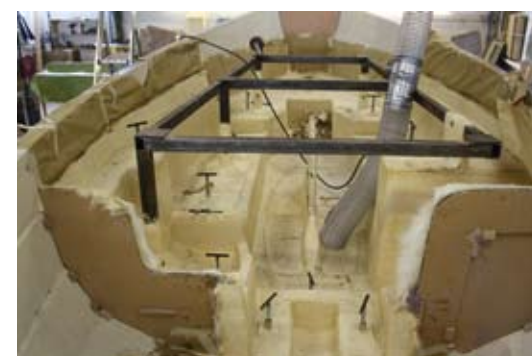
Here the mould has been laid up over the plug. Release plates are fitted and the metal framework is ready to receive the rest of its wheels
