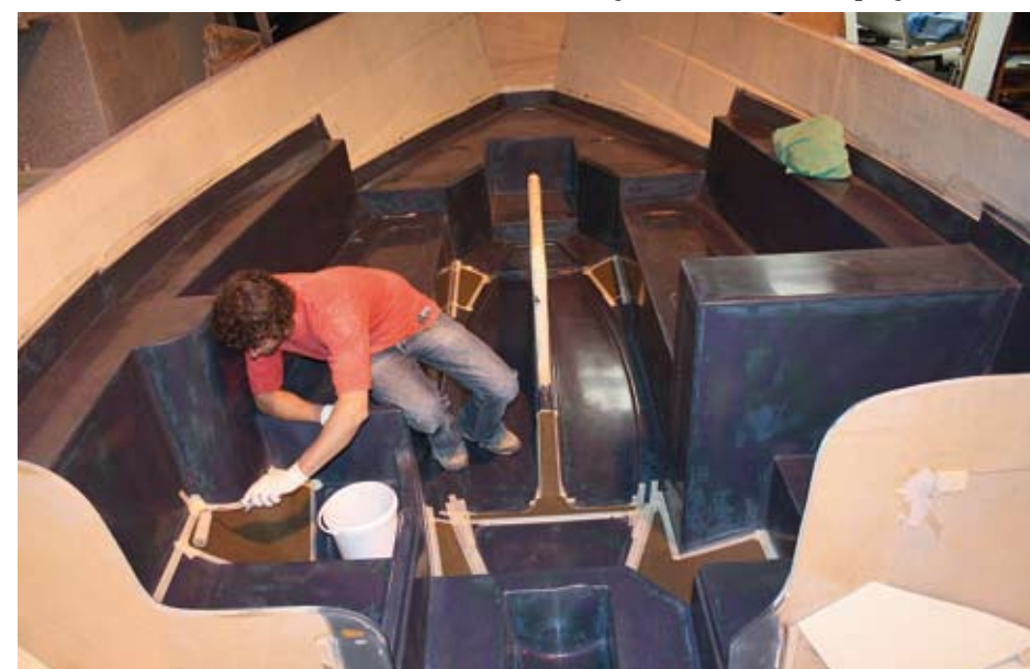
Filled, faired and painted, the plug is nearly complete. A non-slip finish is being applied to angled sections of the cabin sole at the forward end of the saloon and aft by the galley and in the heads
