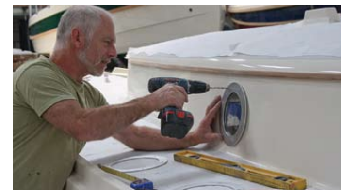
The port holes are suspended with masking tape until their exact positions have been determined. Then it's time to fit them and the rest of the hardware including the stanchion bases. Note the self-adhesive paper applied to the deck and coachroof to protect the gel coat during the fit-out
