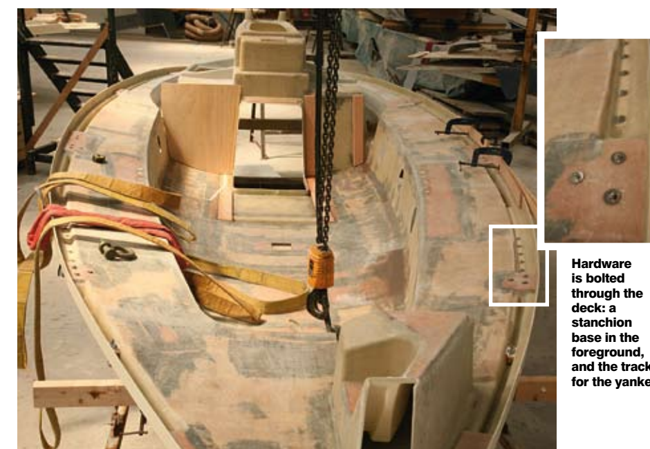
Inside the deck moulding, the plywood and balsa can be seen through the inner laminates. The dark areas are where filler has been applied to ensure an even thickness
